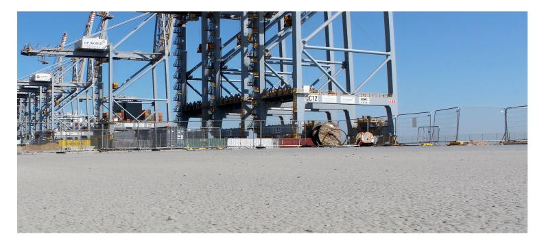
Hardicrete™ consists of an open graded receiving course with a controlled void content, typically laid at a 40mm depth, filled with a resin cementitious grout manufactured by Miles Macadam. It is a flexible, jointless, heavy duty surface course with fuel resistant properties and high load capabilities to minimise rutting or deformation.
